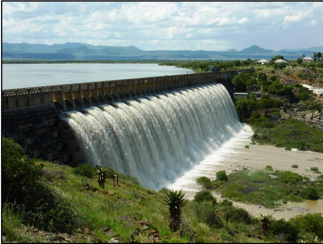
Nqweba Dam overflowing on 11/02/2011
